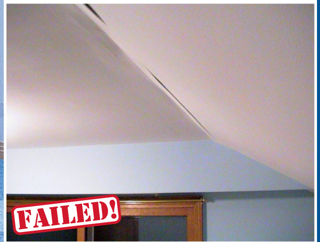
Inside Corners without Expansion Control
